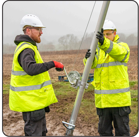
8. Raise the pole by operating the winch and the sheerlegs will become self-supporting due to the weight of the pole on the wire rope.
