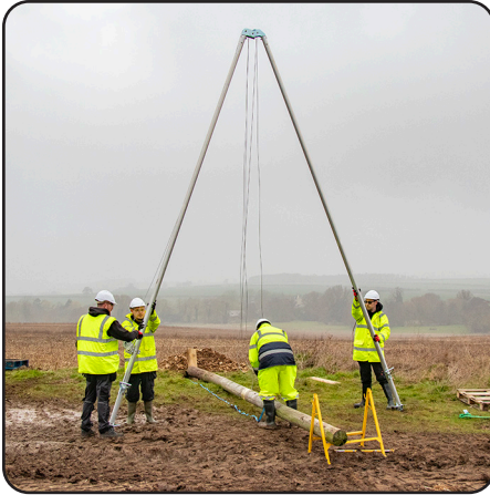
7. Raise the sheerlegs to the vertical and ensure that the feet are firmly based and will not slip as the pole is raised as the sheerlegs lean from the vertical.
