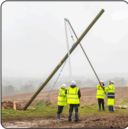
9. As the pole is raised further, the sheerlegs will lean towards the pole hole. When the top of the pole is high enough, the base will slide gently into the hole.
