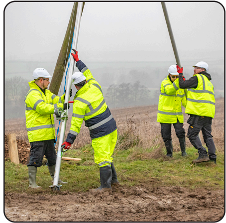
10. Setting the pole. When the base is resting on the bottom of the hole use the handles at the lower end of the sheerlegs to set the pole in a vertical position.
