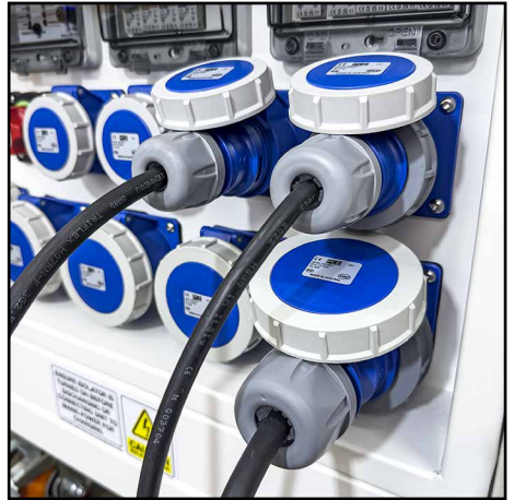
6. Make connections to the relevant outlet sockets and make sure the plugs, couplers and cables are suitable for the loads demanded.
