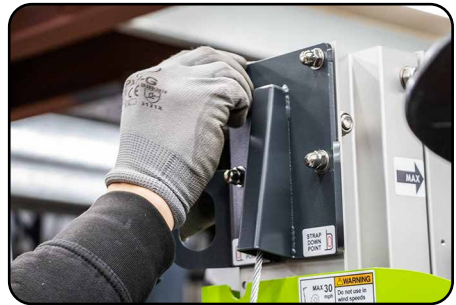
10. Once loose fully remove the nuts and washers, and remove the existing mast wire cover.
