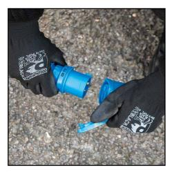
11. Connect the mains input lead to the fitted light head. Observe the local voltage is correct to match the input range of the LED driver (100-277V AC) and switch on / connect power.
